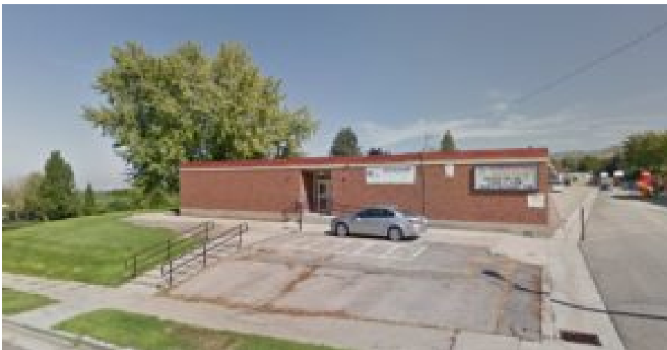
Morningside Elementary School, Holladay, Utah
